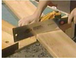
Cut off any bad ends and then cut the boards to length
