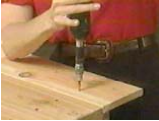
Pre-drill with a counter sink bit and attach the top boards
