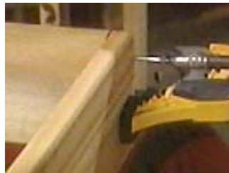
Use at least two screws to attach each corner together
